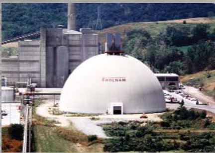
Holcim Cement - Clarksville, Missouri
