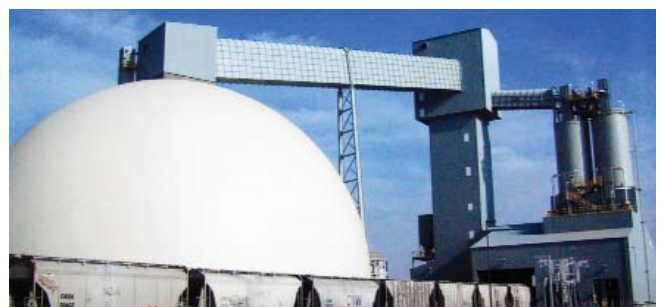
California Portland Cement - Stockton, California
