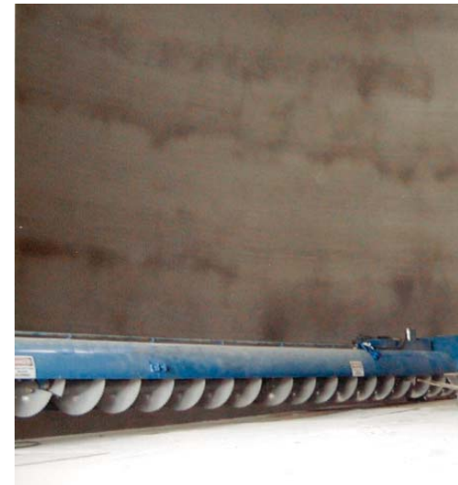
Tubular shaped bridge and screw near
