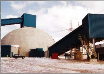
Ontario Power Generation - Ontario, Canada
