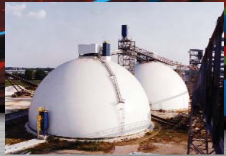
Holcim Cement - Operated by Kinder Morgan - Reserve, Louisiana
