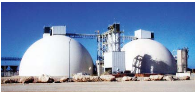
Hawaiian Cement - Barbers Point, Oahu, Hawaii
