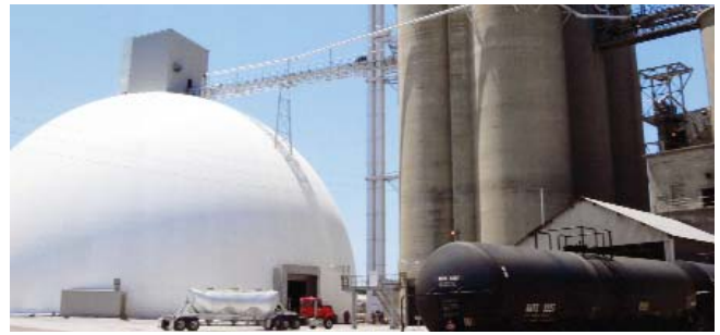
Ash Grove Cement Company - Chanute, Kansas
